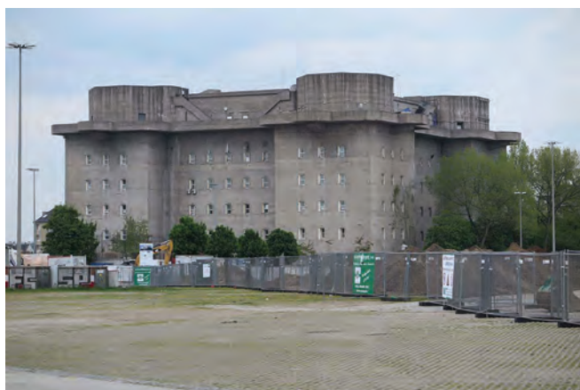
The Flak Tower at Heiligengeistfeld a few hundred metres from our hotel. It can be seen that windows have been inserted post-war to allow for re-use which was apparently part of the original plan
